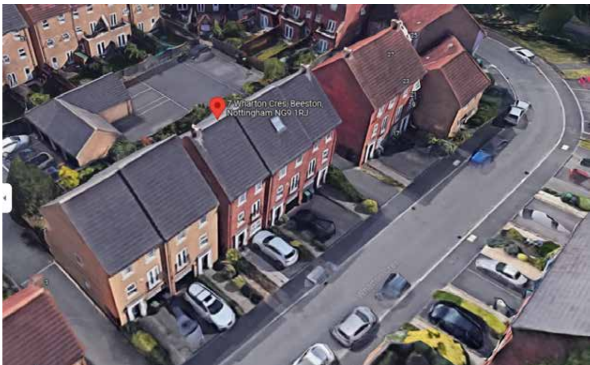
Street scene, with site in centre (Google Maps)
